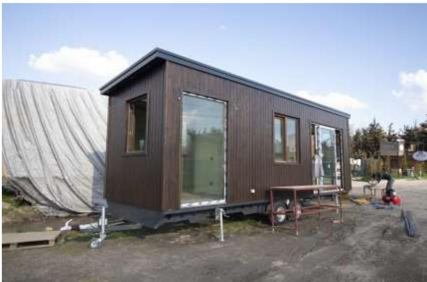
Pic 43 Kiln dried wood facade (vertical flooring)
